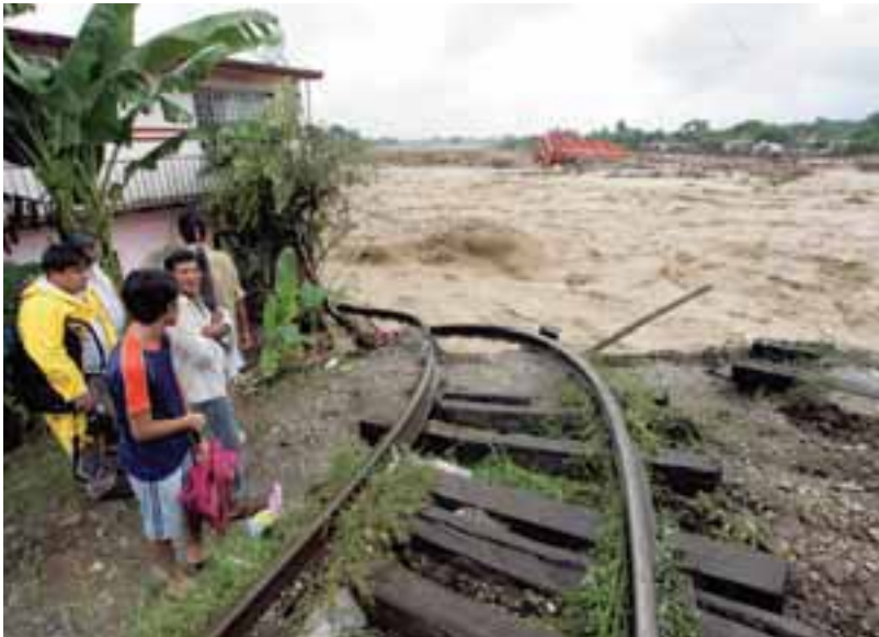
A bridge devastated by natural disaster, Venezuela
