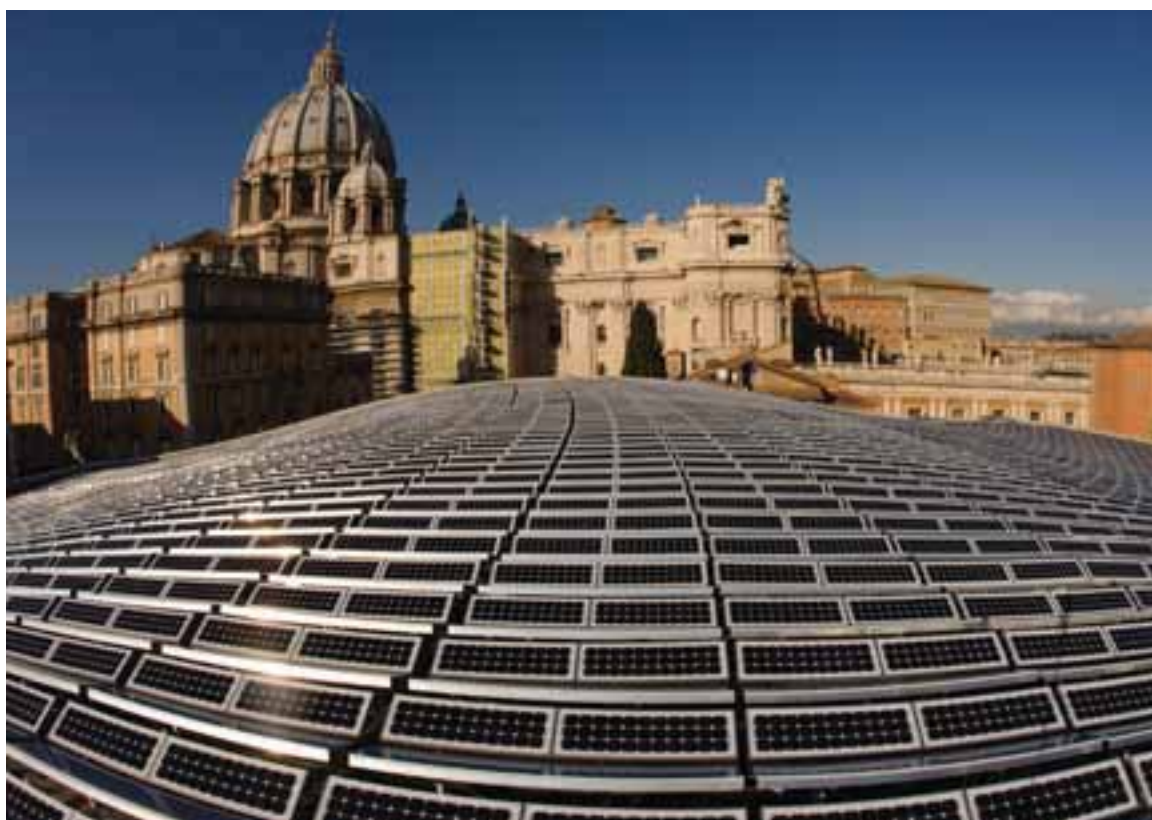
Sustainable buildings: solar panels on the roof of the Paul VI hall near Saint Peter's Basilica, Rome
