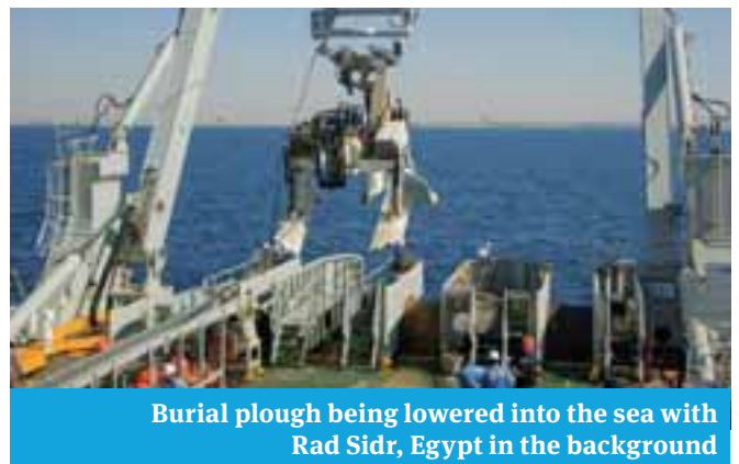
Uraduct installation aboard the CS Tyco Reliance
