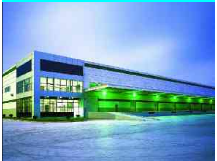
The ProLogis Park Lingang located in the Shanghai Lingang Logistic Park
